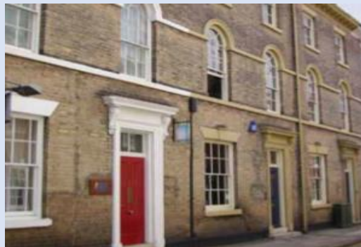
18-28 Friar Lane- Repeated recessed doors and sash windows
