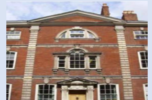
17 Friar Lane- Continued red brick frontage with stone pilasters and arch sashed windows
